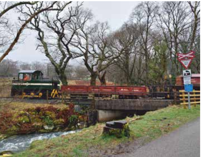
PW train with a DZ and followed by a ballast hopper on relaying work at Cwm Cloch on the WHR. David Firth
