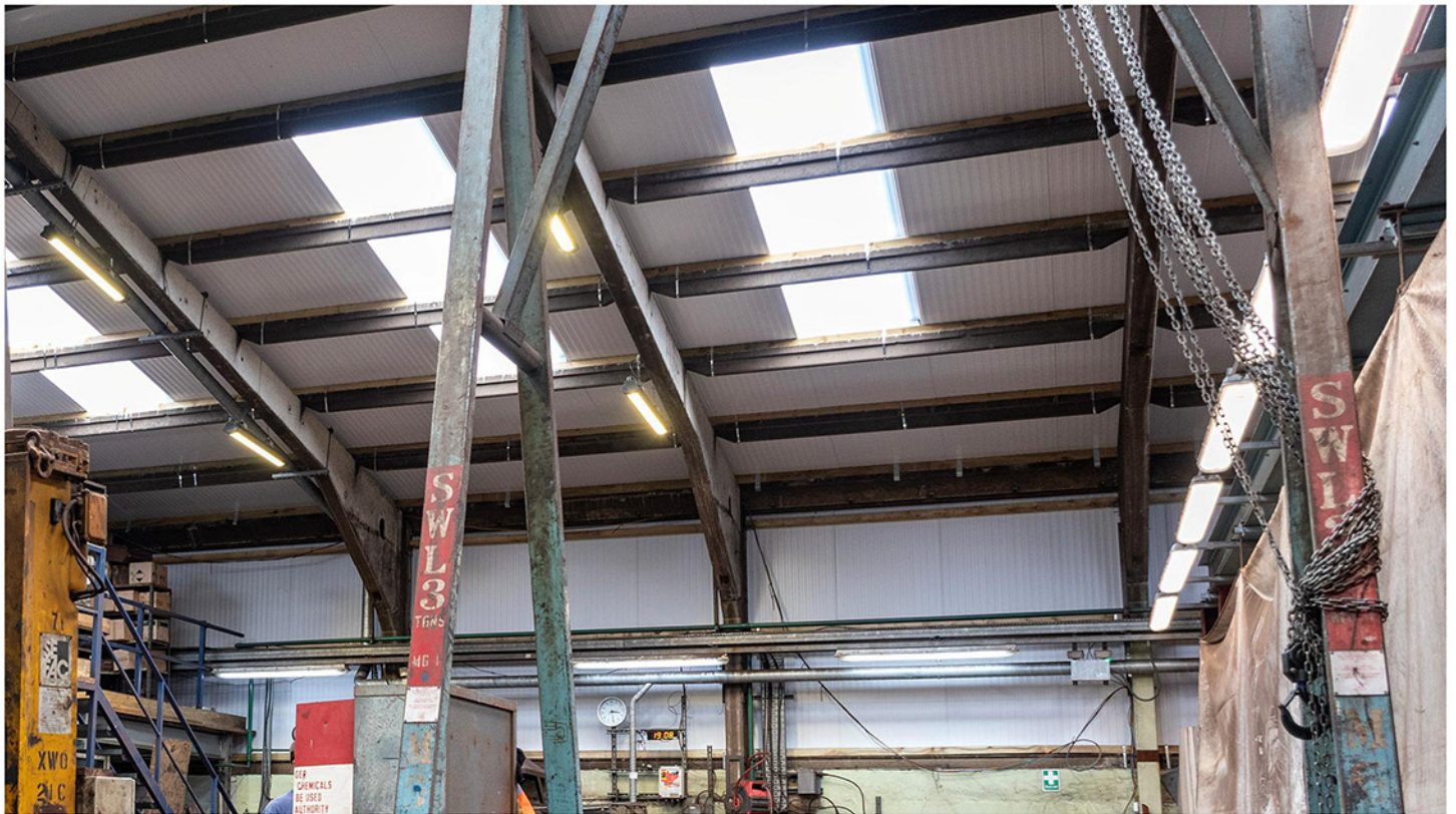
A view of the new roofing panels and skylights installed on the New Erecting Shop. These provide greatly improved working conditions for the staff - with better year-round insulation and enabling more light to illuminate work in progress below. Roger Dimmick
