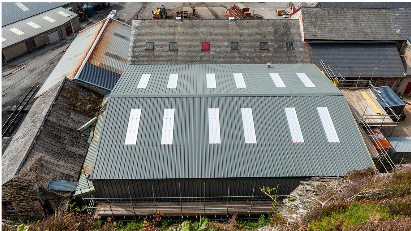
Looking from on top of the quarry face above Boston Lodge, it is easy to see the difference between the 'New' and 'Old' buildings - especially now that the 'New' Erecting Shop has its recently fitted roof and skylight panels in place. Roger Dimmick
