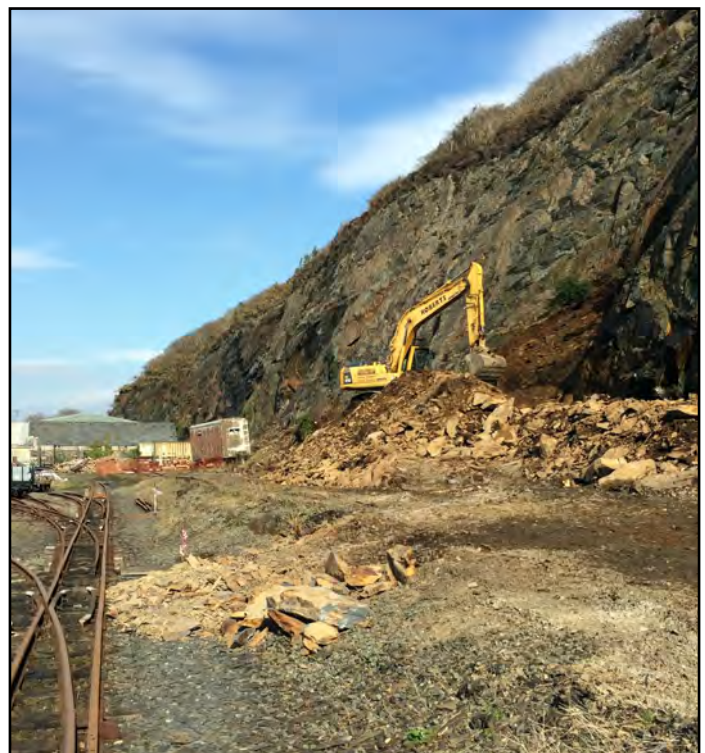
The next stage of the Boston Lodge redevelopment has started with land clearance and levelling at the foot of the cliff to make space for a storage facility to be built in the future.
